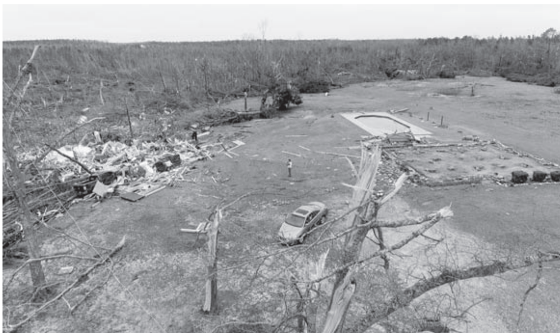
Debris from a home litters a yard the day after a tornado blew it off its foundation, at right, in Beauregard, Ala., Monday, March 4, 2019.
